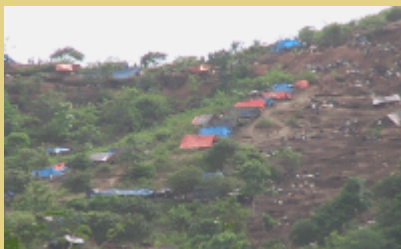
Damage caused by illegal mining at Pondok Ganjar, Selodong, Sekotong, Kabupaten Lombok Barat.
